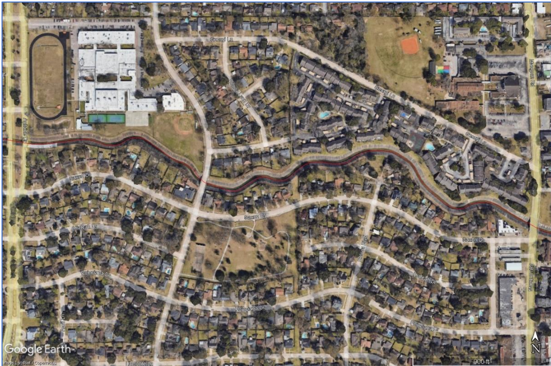
Figure 2: Stretch of the AU bordered by many parks and schoolgrounds. Identified during desktop review as a possible source.
