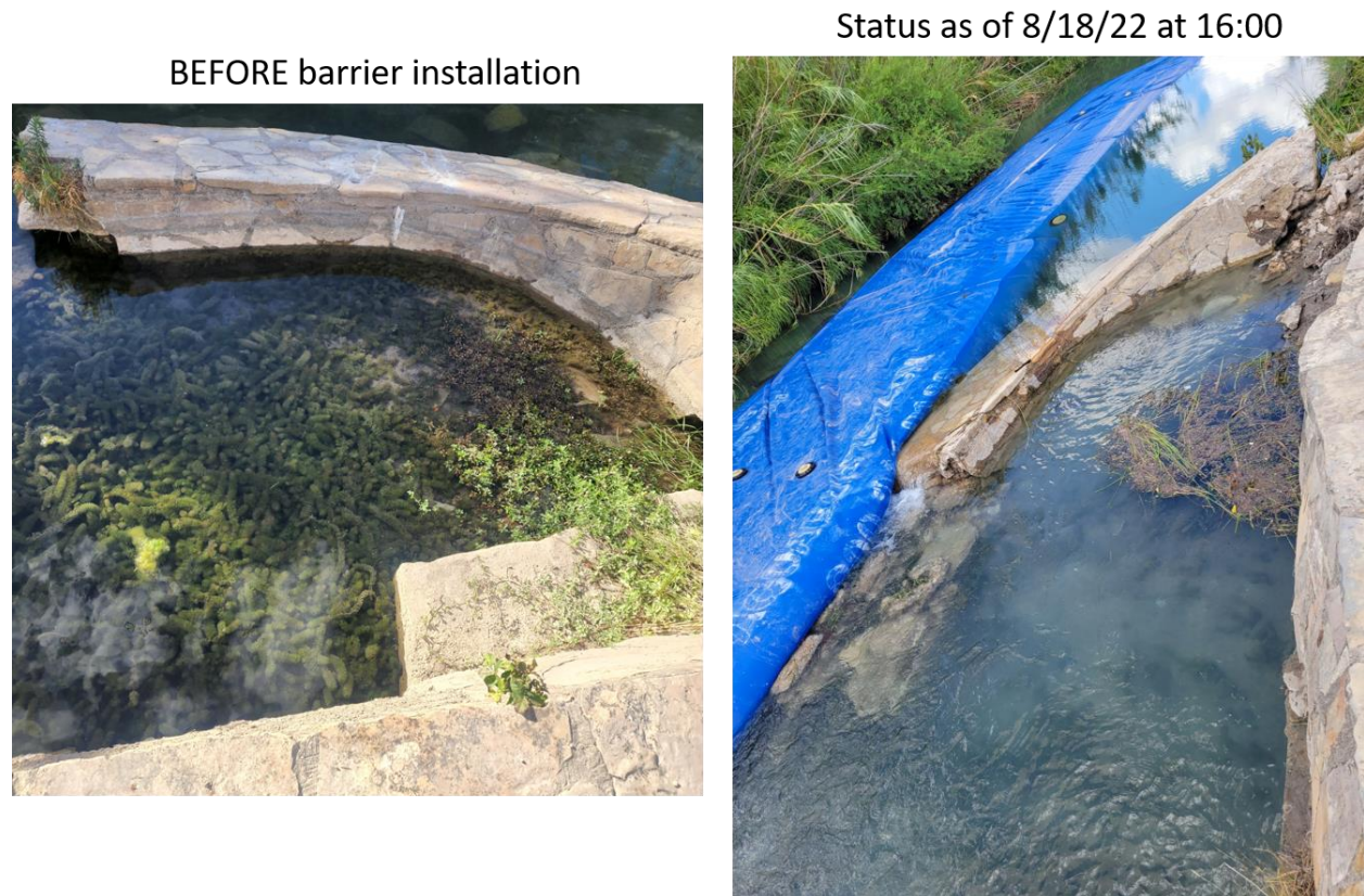
Figure 7 Example of artificially increased water level and flow through confirmed Devils River Minnow ( Dionda diaboli ) habitat due to installation of coffer dam segments on August 18, 2022. Images were submitted in conjunction with USFWS Permittee formal letter to USFWS on August 18, 2022 (Attachment 3). Segment was removed from the channel on August 19, 2022.
