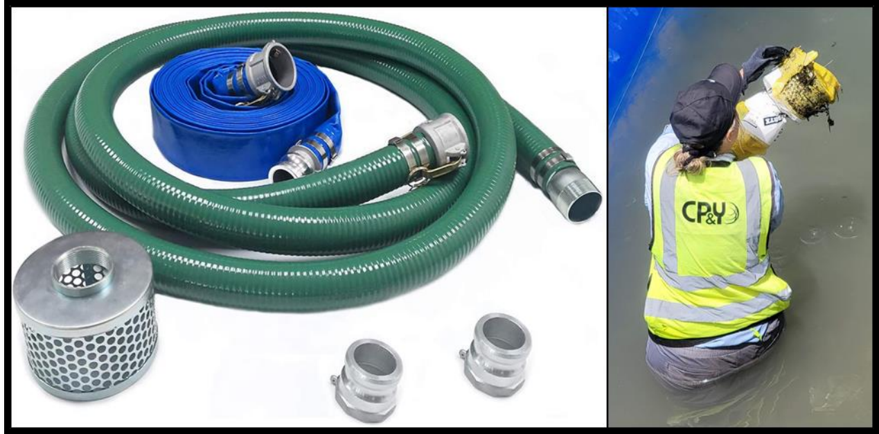
Figure 2 Left image: example of strainer basket (lower left of image), intake hose (green), PVC discharge hose (blue), and quick connections (lower right of image) used for dewatering dammed area. Right image: Biologist removing accumulated vegetation and checking for mortalities on secondary exclusion device around strainer basket (yellow mesh).
