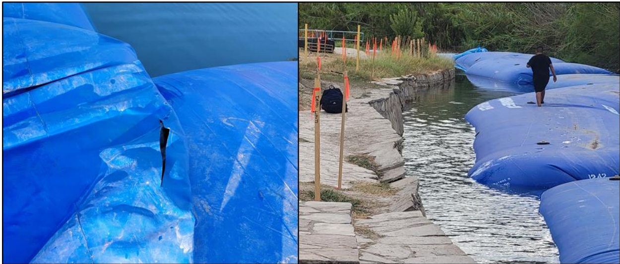
Figure 8 Left image: example of vandalism (laceration) to cofferdam section (observed on August 11, 2022). The laceration was successfully patched on August 11, 2022. Right image: example of public access to and use of cofferdam section(s) (observed on August 13, 2022).
