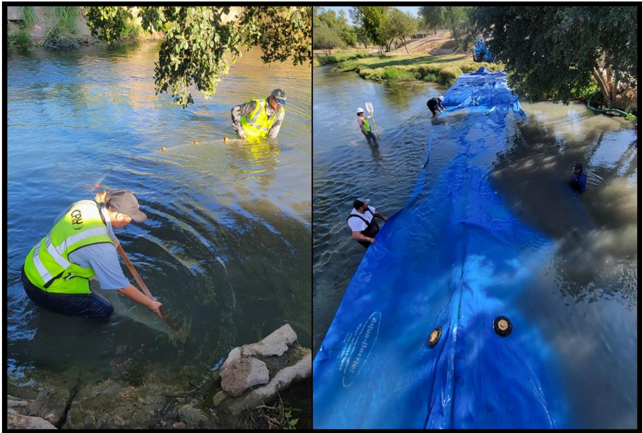
Figure 1 Left image: biologists flushing area prior to in-water construction and dam section installation. Right image: installation and inflation of cofferdam section after area flushing.
