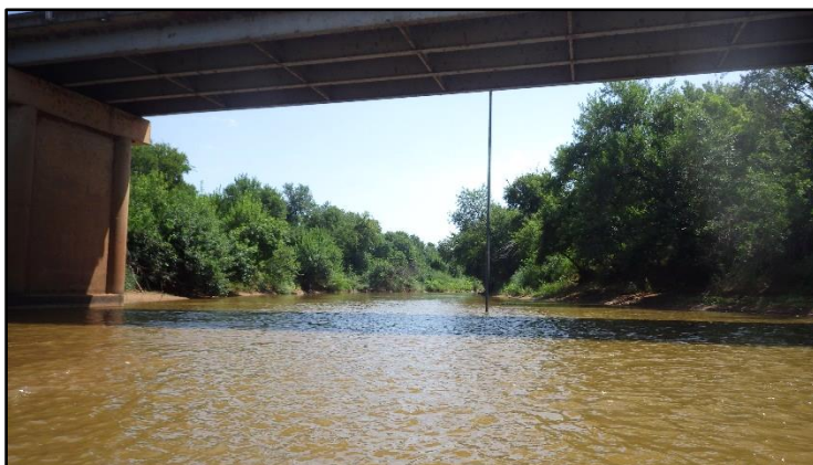
Downstream taken from transect 1 during critical period.
