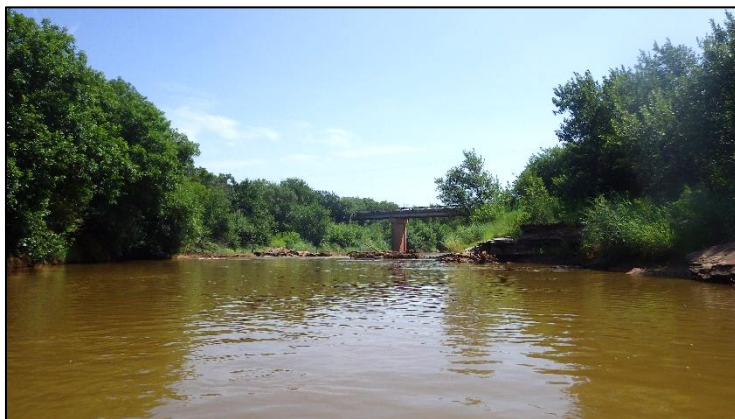
Downstream taken from transect 2 during critical period.
