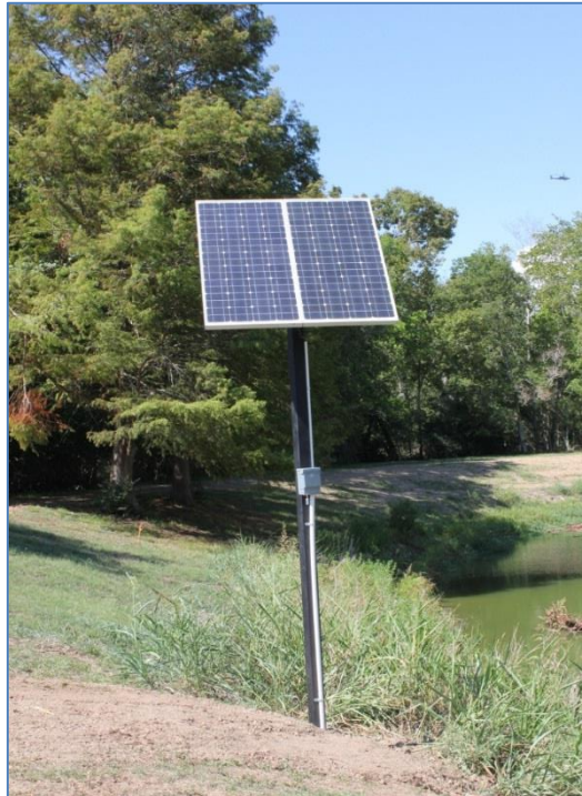
Figure 22. Solar panel that powers a pump which conveys water from Horsepen Bayou uphill to the top of the secondary wetland complex for additional water quality treatment through the created wetland.
