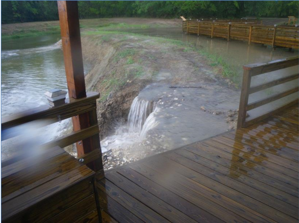
Figure 10. Photo of the Levee breach and erosion experienced by an extreme rain event post-construction at the UHCL wetland into Alligator Pond
