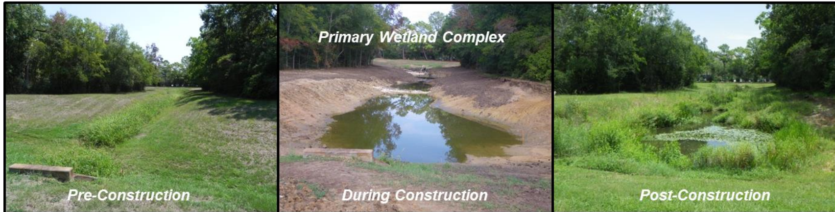
Figure 12. Time series photographs of the primary wetland complex showing pre-construction, during construction, and post-construction conditions.
