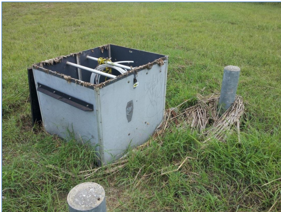
Figure 15. Debris at the high edge of weir 2 observed on June 31, 2012 between pond 2 and pond 3 believed to have been deposited by flood events.
